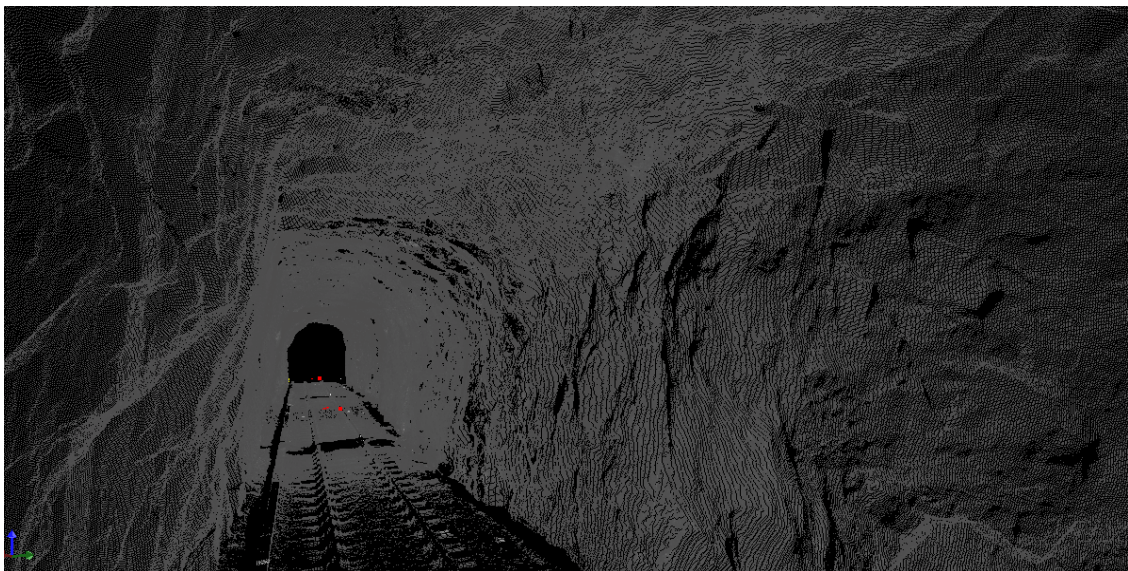
Figure 24. ScanTech point cloud data processed with Pointools of the Ffestiniog Tunnel.
