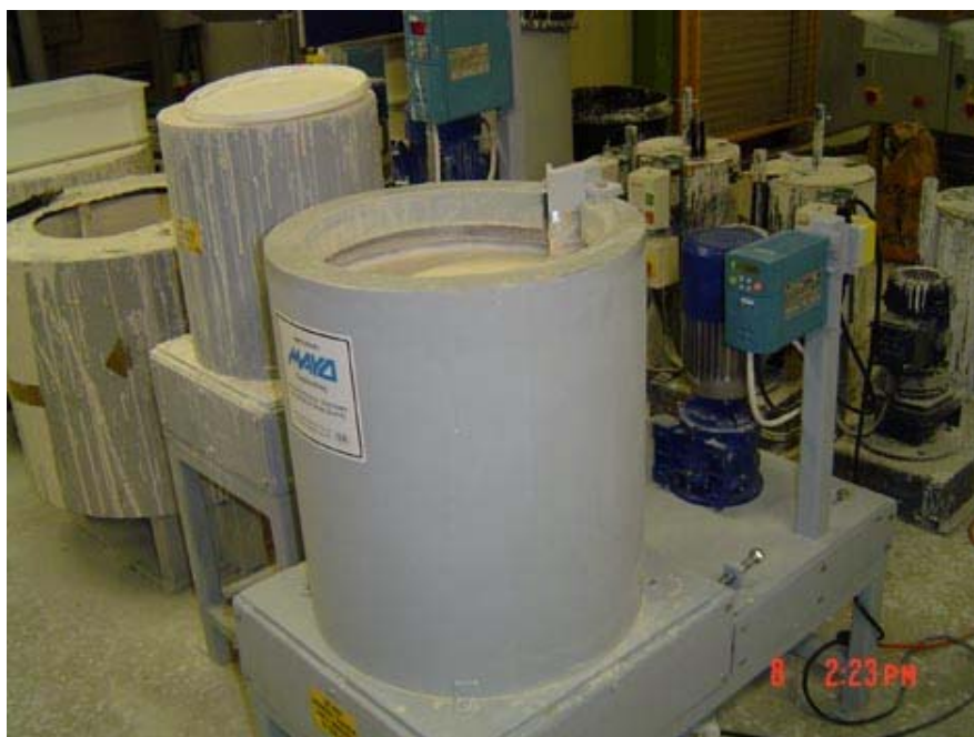
Figure 4: Slurry mixing tank.
