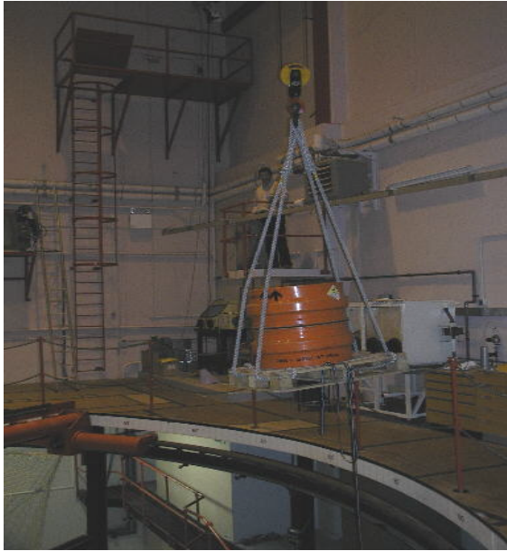
Figure 2-2: Lowering the drum to the bottom of the Pit
